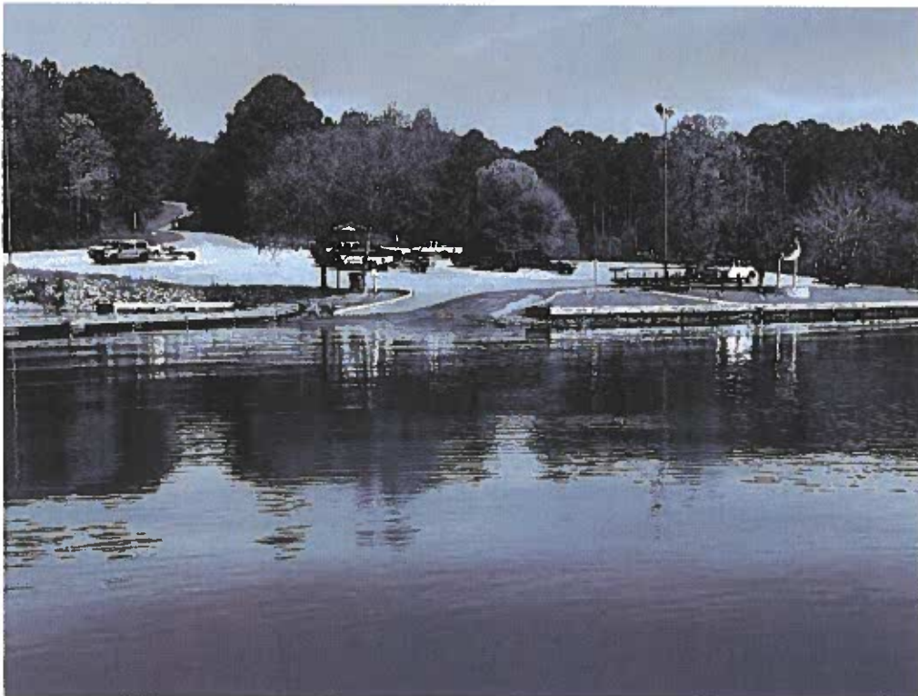
Figure 4: Boat Ramp, Pier, Float, Boardwalk, and Rip-Rap
