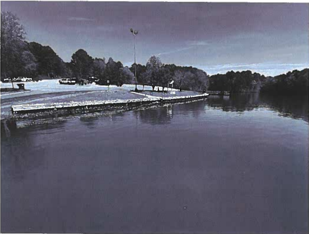
Figure 6: Boardwalk and Pier
