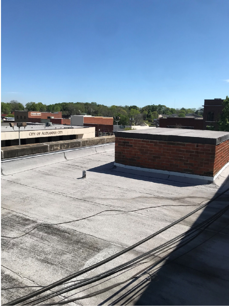
Picture #15. Roof of police department
