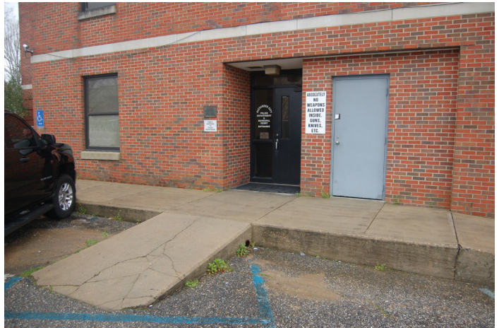
Current ADA Entrance
