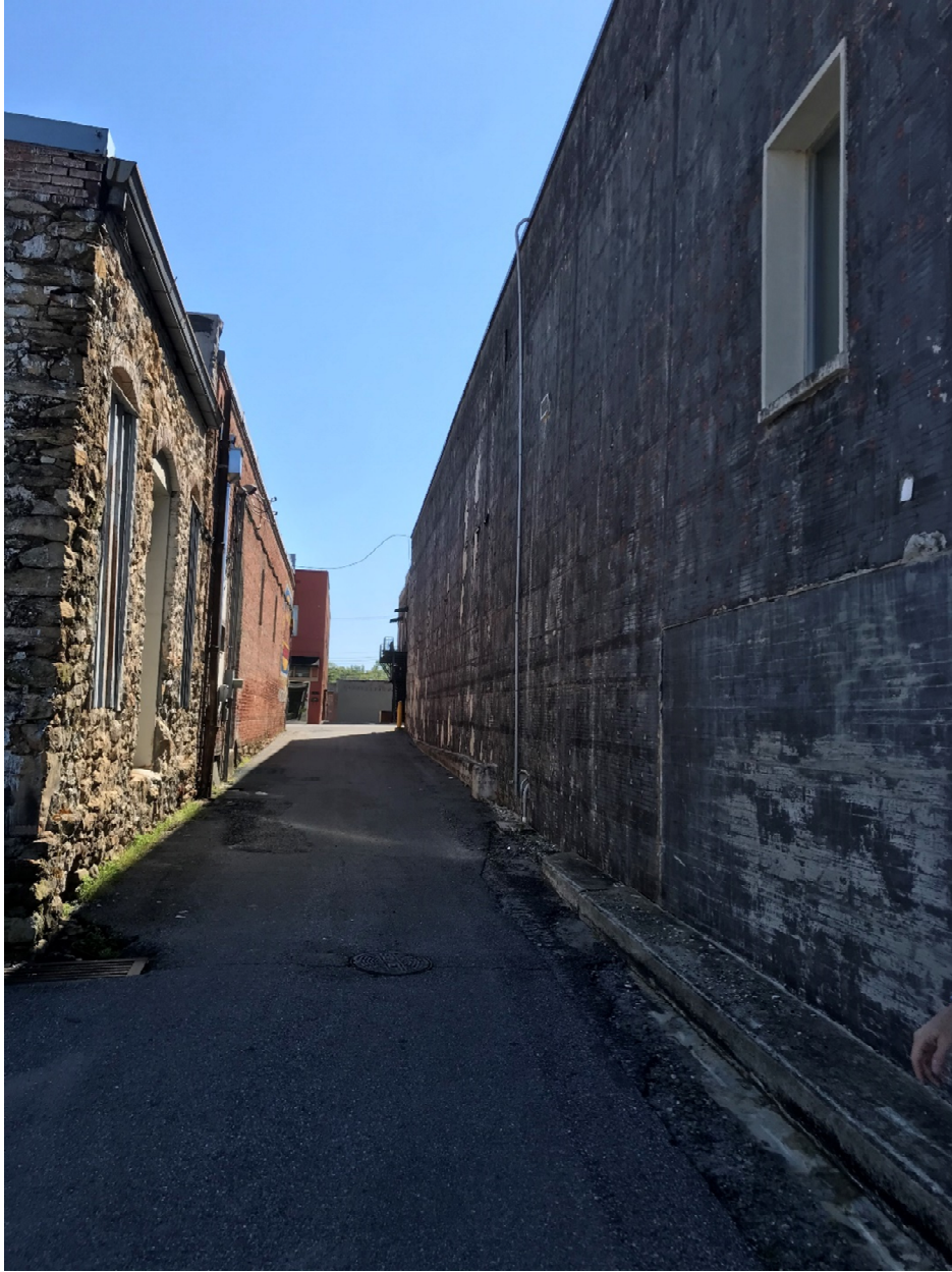
Picture #8. Exterior finish has been removed
