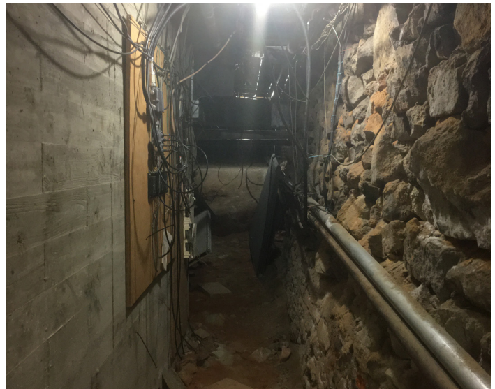
Stone Walls in Crawlspace
