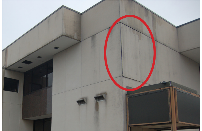
Movement in Pre-Cast Panels
