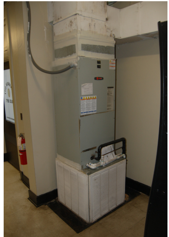
Free Standing Mechanical Unit with Corridor Return Air
