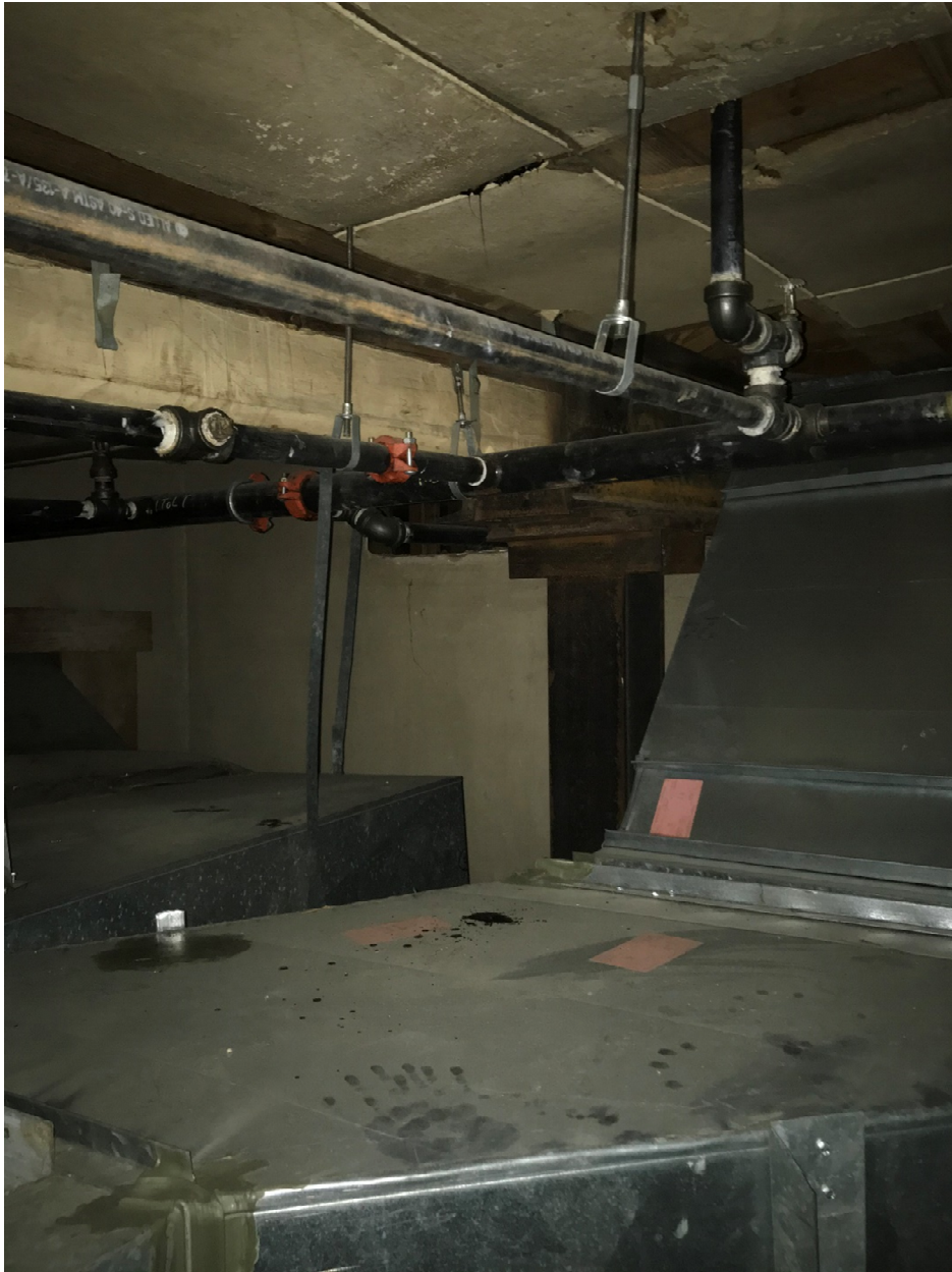
Picture #7. Added steel most likely from an addition
