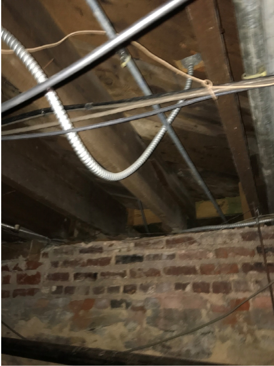
Picture #3. Wood framed floor system
