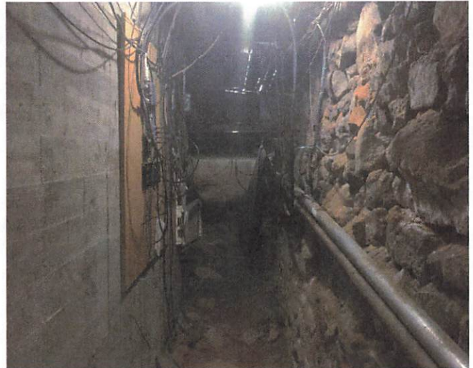
Stone Walls in Crawlspace
