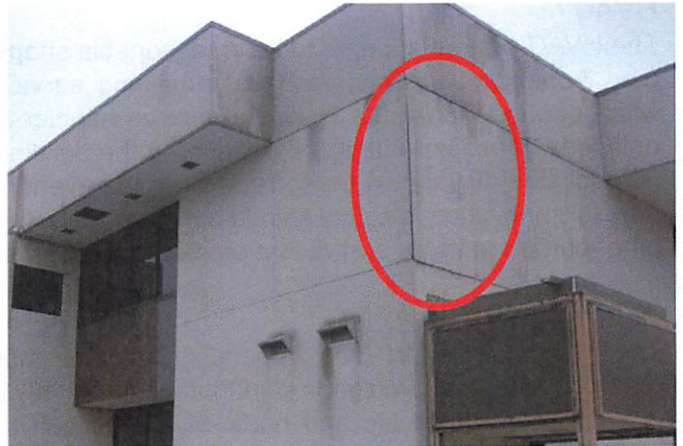
Movement in Pre-Cast Panels
