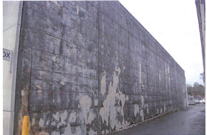
Exposed Wall Substrate where Stucco Removed
