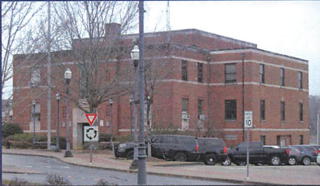
Police Department Building
