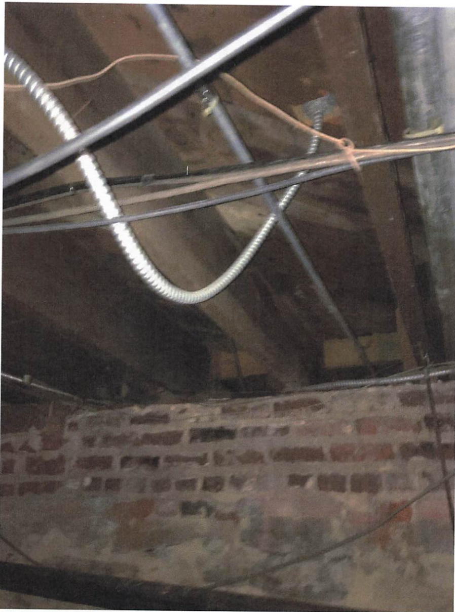
Picture #3. Wood framed floor system
